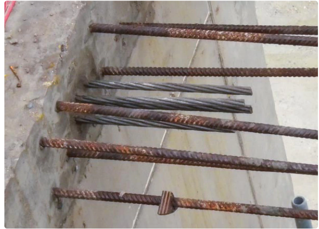
2. Post-tensioning tendon ducts
