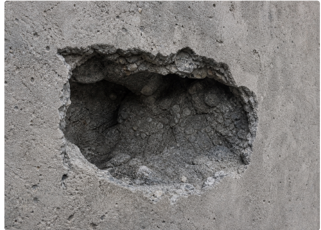
2. Internal voids and cavities
