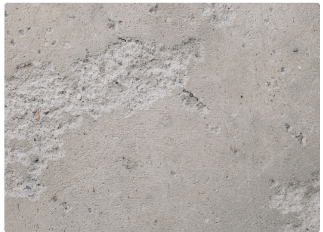
4. Freeze-thaw damage
